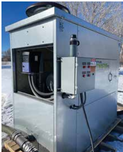
Titus Twister FL (Floating Aerator) control, power and air supply unit on the shore of the St. Stephen's School Wastewater Treatment Lagoon.
